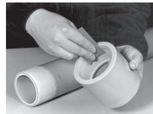
Abrade pipe and socket
