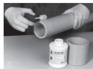
Apply solvent cement to the outside of the pipe
