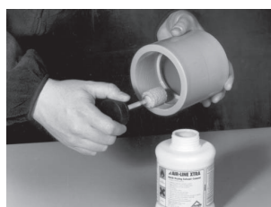
Apply solvent cement to the inside of the fitting
