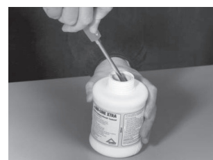
Stir solvent cement
