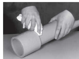
Wipe off excess solvent cement
